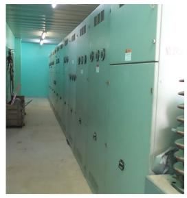
Figure A-3: WAL Substation 12.5 kV Switchgear Rear Layout
