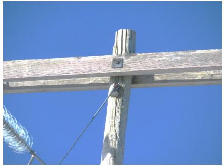
Figure B-11: Deteriorated Pole Top
