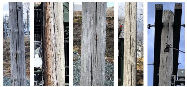
Figure B-3: Deteriorated Wood Poles
