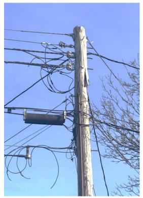
Figure 3: Deteriorated Secondary Pole
