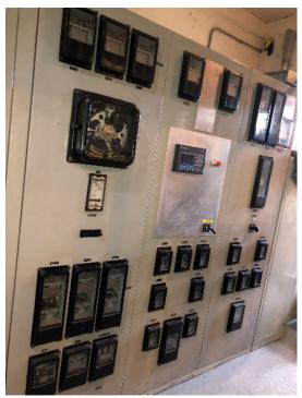
Figure 7: Electromechanical Protective Relaying
