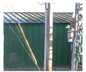
*Figure A-8: WAL Substation Building Roof Showing Signs of Deterioration*
