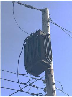
Figure 4: Deteriorated Pole and Vintage Transformer
