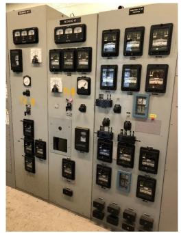
Figure B-6: MOL-T1 and MOL-T2 Protection Equipment
