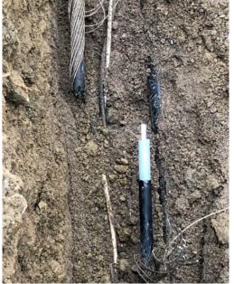
Figure 2: Loop 34 Primary Conductor Failure Repair
