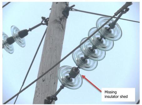
Figure B-7: Broken Insulator Shed
