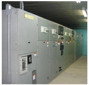
*Figure A-2: WAL Substation 12.5 kV Switchgear Front Layout and Protection and Controls*
