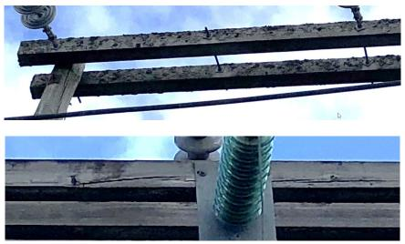
Figure B-4: Deteriorated Wood Crossarms
