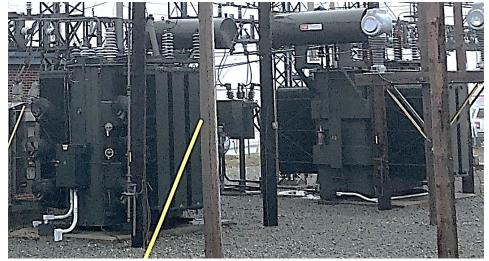
Figure B-2 shows the MOL-T1 and MOL-T2 transformers.
