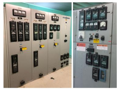
Figure A-6: Electromechanical Relays
