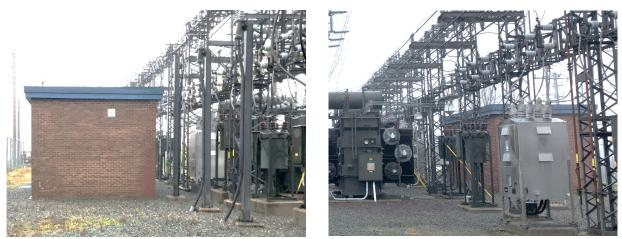
Figure B-8: MOL Substation Control Building with Insufficient Clearances to 12.5 kV Structure
