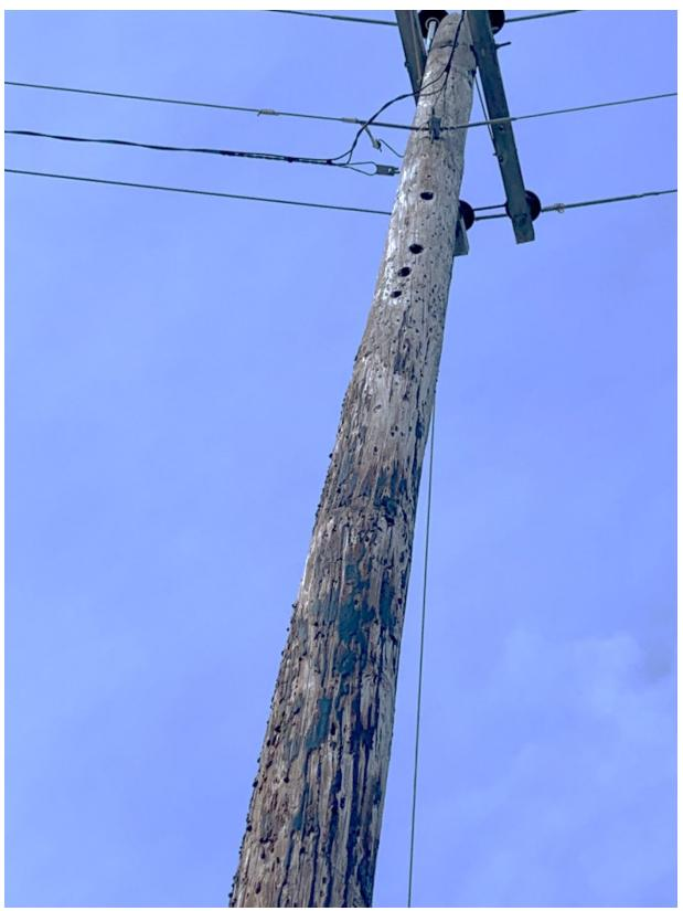
Figure C-4: Deteriorated Pole with Woodpecker Holes
