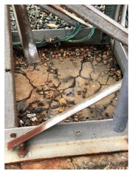
Figure B-5: Deteriorated 12.5 kV Concrete Pier Foundation
