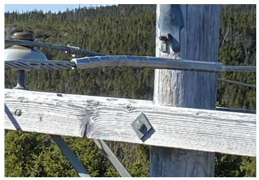
Figure 4: 2/0 ACSR Conductor Repair
